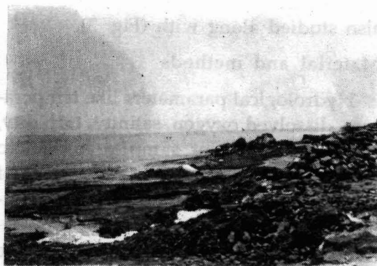
Fig. 2. The ash laden water escaping through dyke into the sea.
